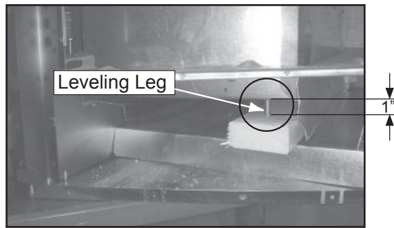
Figure 11.1. Ensure that the leveling leg is positioned over the support material before leveling the insert. If using combustible material for support a minimum 1" airspace is required between the insert and the combustible material.
