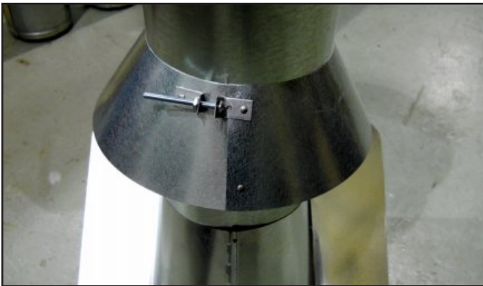
Figure 7.14 insert Bolt into Brackets
