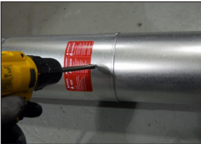
Figure 7.4 Screws into Slip Section
